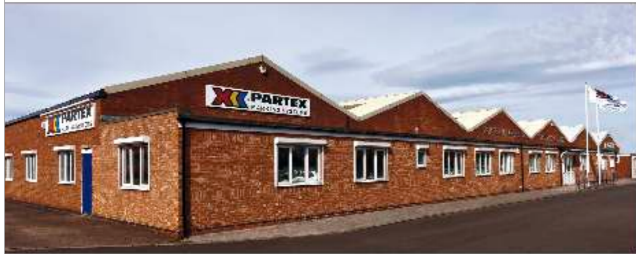
Partex UK headquarters
